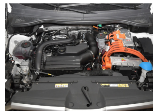
Orange-coloured cables in the engine compartment
